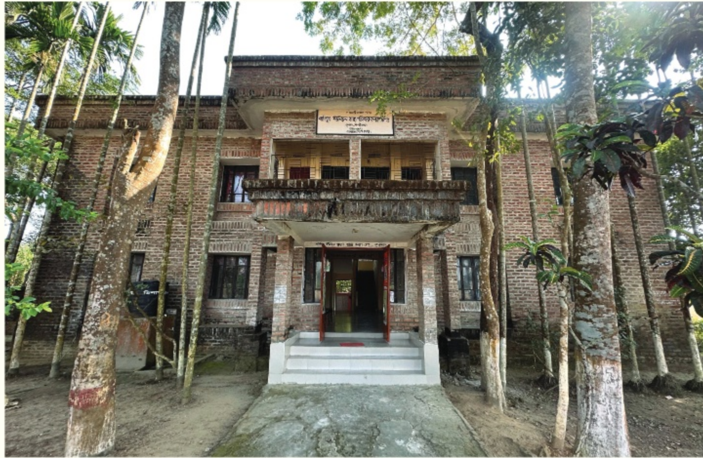
The Health and Family Welfare Center building at Kadipur union, Kulaura.
